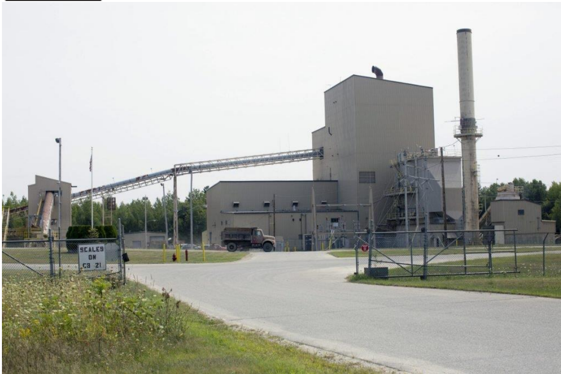
Stored Solar LLC received a $1.2 million state subsidy intended to keep its wood-fired power plants operating and their workforces intact in the Penobscot County town of West Enfield, above, and the Washington County town of Jonesboro. Staff photo by Brianna Soukup
